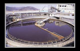
This technology delivers a range of commercial and environmental benefits to Sewage Treatment Plants (STP's). It binds heavy metals into non-bio-available forms, removes phosphorus and odor from sewage effluent and reduces Biological Oxygen Demand (BOD) and Total Suspended Solids (TSS) in the effluent stream, and treats bio solids for pathogens, odor and other contaminants, while maintaining a stable pH.
